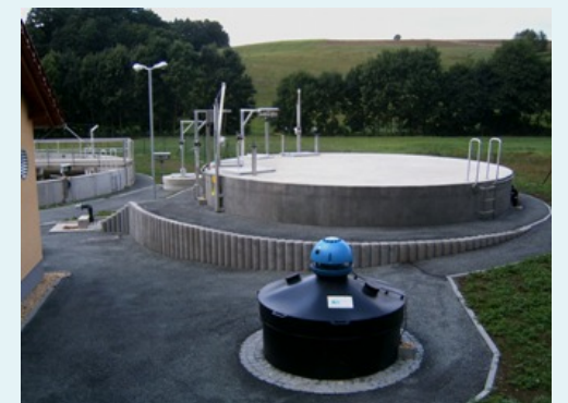
BEGA system used to empty a pressure pipe end sump and screening channel
